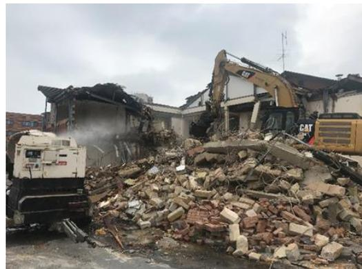
This sequence continued until the building was demolished. All waste was separated during the demolition, ready for disposal at registered recycling facilities. The concrete and bricks were retained on site and crushed using Lawson Group's own mobile crushing equipment.
