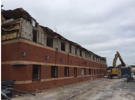
A 360-excavator was used with a hydraulic shear attachment. The roof was removed back to the first supporting column allowing one bay of the roof to be lowered carefully to the 2nd floor slab.
