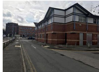
white panels were made up of asbestos cement sheeting. A live substation was located within the site, which was planned for reuse, so the works included its protection. Service access to the Zurich Tri-Centre office was required through the site perimeter. This redundant building had been used for emergency temporary homeless accommodation over a cold period. A full needle sweep of the building was required before works could commence.
