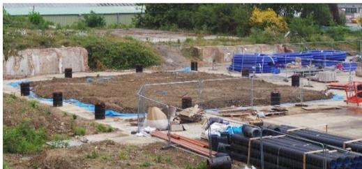
Japanese knotweed was found behind the canteen and 80-tonnes of material were dug out. This contaminated topsoil was laid out up to 300mm thick on 1,200-gauge polythene sheeting. This material was left on poly sheeting for a three-year quarantine period (possibly five years) - depending on evidence of regrowth or only when the inspectors were happy that all the spores and plants had disappeared.
