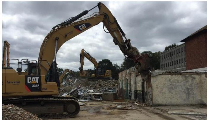
Internally, this building was a challenge. Soft stripping was needed, and tiles needed to be removed for a bat check before any works could commence - but no bats were found in this building. A CAT scan of the site was carried out by the demolition supervisor who had received the relevant cable detection training.
