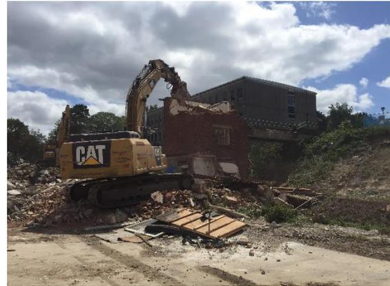
walls. This process was repeated until the entire building had been deconstructed. The concrete and brick access bridge was also removed. The wood, brick, concrete and other associated materials were removed and lowered to ground level away from the building. These were processed in accordance with the method statement devised by Lawson Group's highly qualified project management team.
