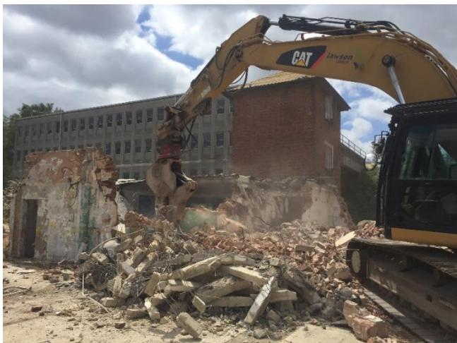
After completion of the soft strip, demolition could commence. This started on the structure located at the lower level. A Lawson Group owned CAT 336F excavator, fitted with a hydraulic grab attachment, was used to dismantle the concrete and brickwork structure. Starting from the east-facing side of the structure, the walls were carefully removed, leaving the brick-built tower structure.
