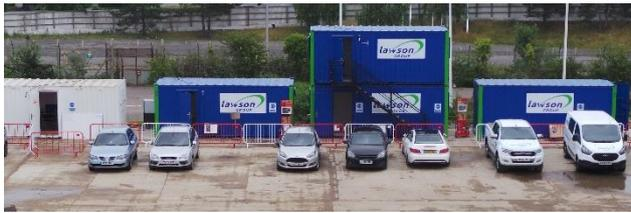
Site welfare and parking were located on the concrete slab at the front of the site. Heras fencing was supplied by Lawson Group with debris netting attached and was positioned around the boundary of the site. For safety and security, the access gate
