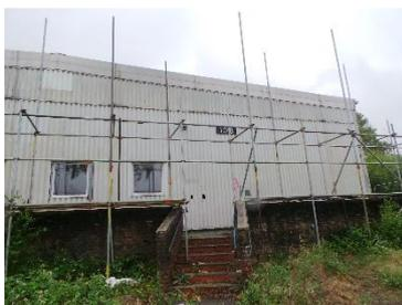
The scaffolding would need to be screened with Monarflex sheeting and required one boarded lift and a loading bay to the back of the building. This would enable the Negative Pressure Units (NPU's) to be positioned on the scaffolding.
