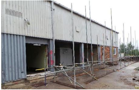
The enclosure would be accessed via an airlock fixed to the external side of the enclosure. Negative Pressure Units (NPU's) would need positioning at the opposite end of the enclosure to the Airlock, on the first lift of the scaffolding. Waste would need to be removed via bag lock and a designated waste route to the enclosed skip.
