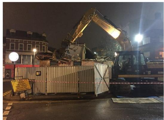
building footprint for the excavator to track on. The external walls of the building were removed last, this, along with a Dust Boss, helped contain any dust generated.
