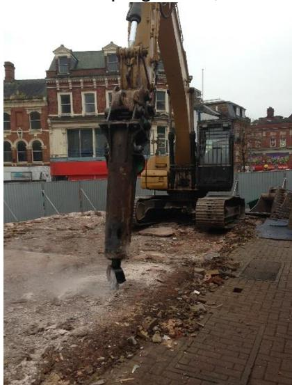
Starting at the edge of the building's slab and at the furthest point away from the site entrance, an excavator with bucket attachment lifted the slab in large pieces. The floor slab and foundations of the building were removed down to 240mm below existing ground level. Next, the footprint of the building was levelled and tracked in. The area was then covered in tarmac, which was managed by Lawson Group.
