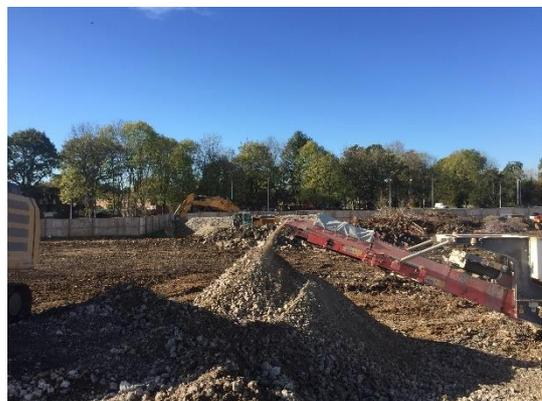
or loading shovel. The discharged material was allowed to heap up to reduce the height the crushed material could fall; this reduced the dust generated from the discharge belt. The crusher moved along the stockpile as and when required.
