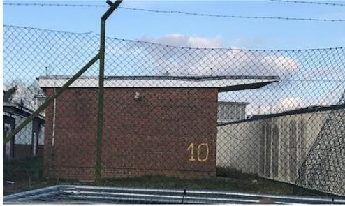
This was a small structure which was demolished using a 360 excavator from the side and working from the top down.
