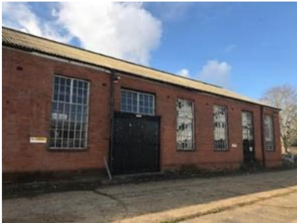
This building had Asbestos roof sheets which had to be removed before the building could be stripped and demolished.
