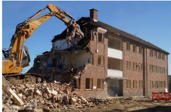
A CAT 323 worked through the demolition arisings to process the materials ensuring that Lawson Group's recycling targets were met. Building 62 was predominantly made out of brick and concrete which was able to be crushed on site with some of the material being recycled as a subbase for the roads.
