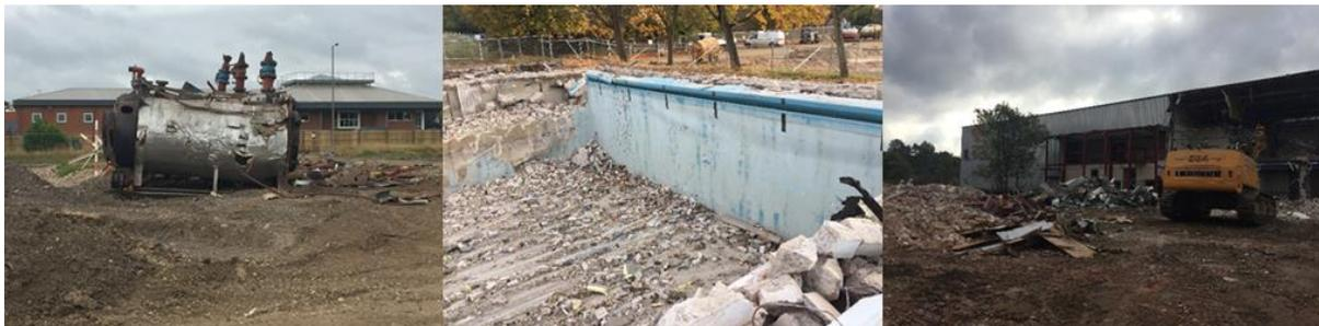
**Building 41** - A sheer attachment on the CAT 336 was used for sorting the demolition arisings from the demolished building, as shown below.
