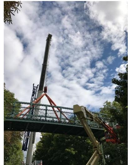
As the final bolts were being cut, the slinger was in contact with the crane operator making him aware of what was happening, and the full control of the bridge was under his command. A tag line was secured to the bridge and used to help control the swing and direction of the bridge. The crane then slowly lifted the bridge which was then lifted up and away from the crane.
