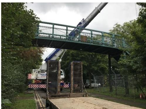
Lawson Demolition operatives then clipped onto a secure structural member using a harness at all times during this working at height stage. Once set up, the chains were checked and were
