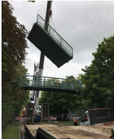
A truck then reversed onto site and parked near to the bridge ready to be loaded. Once the landing was free the crane lifted the sections and slew them onto the waiting truck and trailer.
