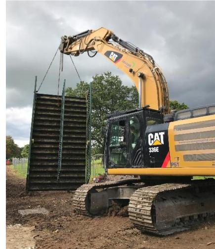
Once deemed safe to do so, the excavator lifted all the concrete out of the ground. For footings that were too large to lift out, a breaker attachment was placed on the machine to break up the concrete first.
