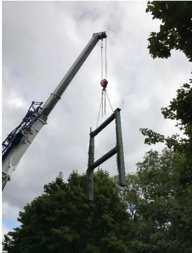
Back on Biggs Lane, the holding-down bolts were cut from the concrete base, once removed, the crane lifted the bridge supports using the same method as before, placing onto the waiting lorry.
