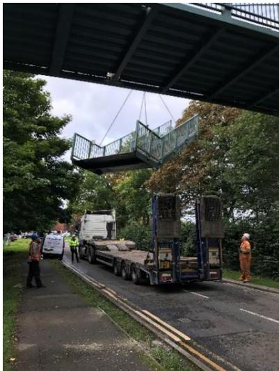
Using the tag line, the bridge was turned ninety degrees and lowered down onto the waiting lorry. Once the bridge section had been placed on the trailer, the load was made secure and then transported around to another area within the Arborfield site. The chains were left on the bridge so it could be lifted off the lorry.
