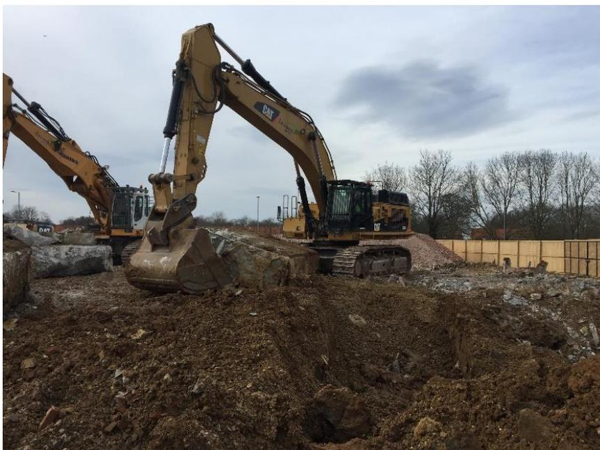
**RESULT:** All concrete hard standings were removed, and all concrete arising's crushed to a 6f2 specification, material permitting. Brick was crushed to a 60mm down crusher run and stockpiled on site. The site was successfully and safely deconstructed ready for the next phase of redevelopment.
