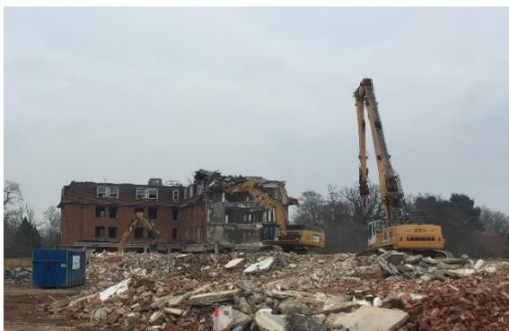
Utilising a High Reach 360° Tracked Excavator with a hydraulic pulveriser attachment rather than a percussive attachment in order to reduce noise and dust emissions, deconstruction of the Sergeants' Mess main building began, The methodology dictated that a top down process was used, removing timber, steel, concrete roof structures for processing and recycling.
