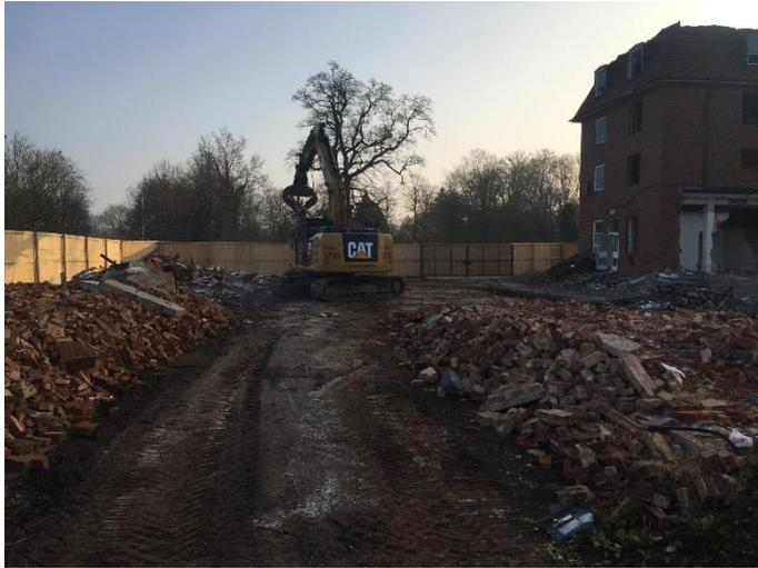
Arising's generated from the demolition were utilised to form a ramp for the excavators to use as a work platform during the demolition of the plant room and remaining high level lift motor rooms and stairwells.
