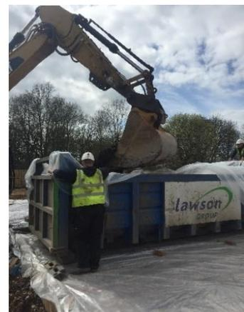
potential spores lying in the soil. All waste was placed in the polythene lined skip which was sealed before removal. All plant and equipment were thoroughly decontaminated following the process. Once this had been completed, the construction of an asphalt covered car park could begin by Lawson Group's team.
