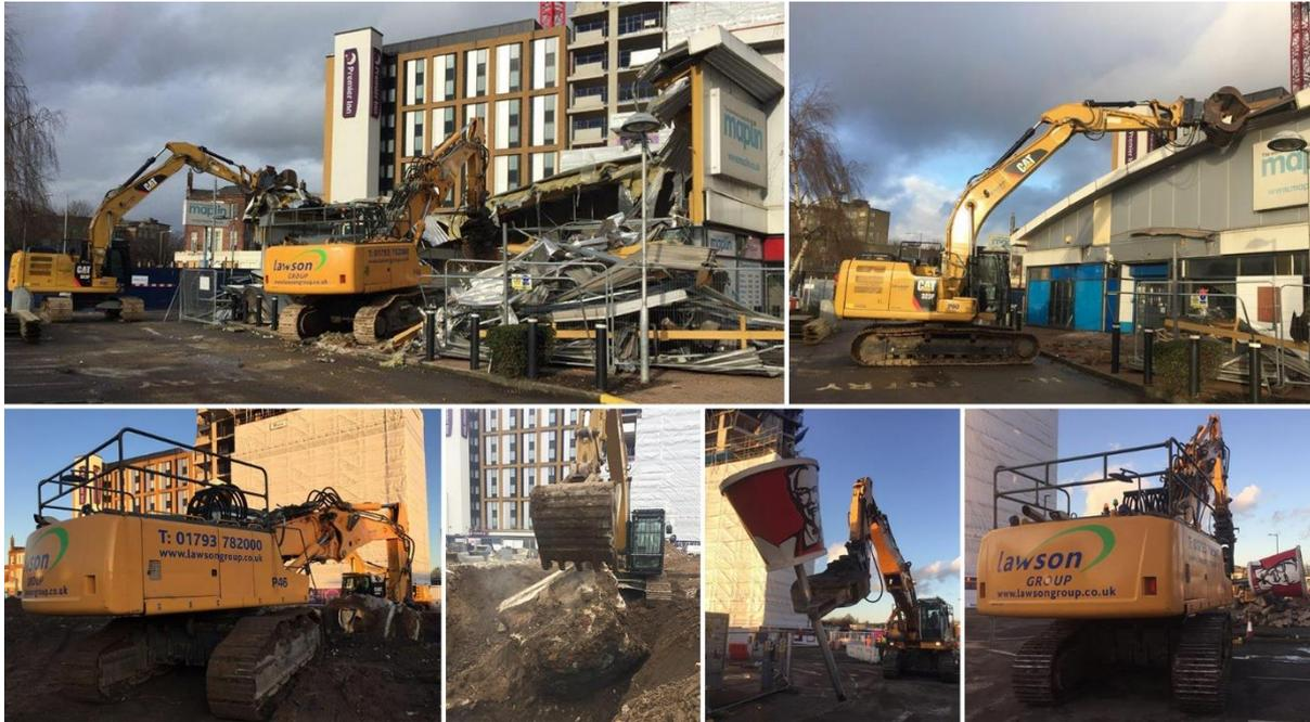
The excavator with bucket attachment then proceeded to lift the slab starting at the edge of the site. The slab was broken into pieces of no bigger than 500cm wide. The slab was stockpiled in different areas ready for removal from site. Foundations of the building were lifted out and stockpiled ready for breaking. This area of ground from, where the foundation has been removed, was then backfilled and tracked in. This process was repeated until all the foundations had been removed.
