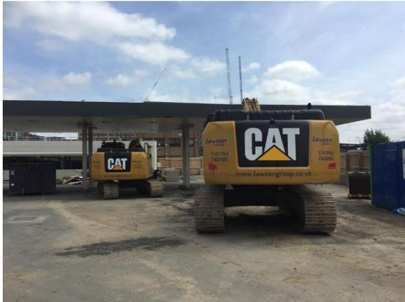
One of Lawson Group's very own 360° demolition excavators, with shear attachment, was positioned at the rear of the garage canopy. All tin sheeting was removed to ground level which in turn exposed the steel frame.
