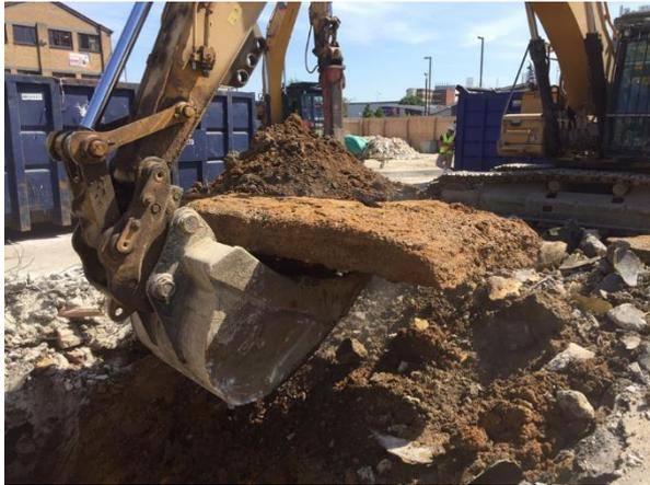
An excavator with bucket attachment dug around each interceptor, a breaker attachment was used to break out the surrounding concrete. Once the tanks and concrete had been removed, an inspection of the area was made by the supervisor. Any suspected contaminated ground was also dug out and stored on plastic sheeting. Once all the concrete had been removed, the sides of the hole were battered back, crushed material was placed in the hole and compacted in layers using a twin drum roller.
