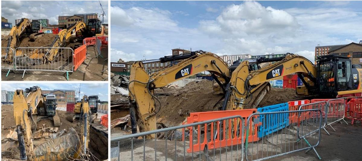
During the above processes, the site manager checked for any signs of contamination within the concrete and soil. After the tanks had been removed, the excavations were stepped back in one-metre high sections. Now all the tanks had been removed, the area was backfilled in 150mm layers using crushed material that was imported.
