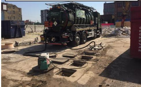
commenced, all the pipework was pumped, washed and given a gas free certificate by the appointed contractor on site. Each tank was dug around and exposed. Using a breaker attachment, a long split was made in the top of the steel tank then a second excavator was used to pull open the top of each tank. A breaker attachment was then used to break up the concrete inside the tank. As works progressed the supervisor monitored the removal.
