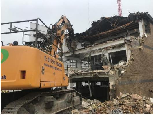
from the roof was removed by a second excavator. As each bay was removed, the side walls and windows were lifted down using the grab attachment. Like the first three buildings, the internal floors of this building were removed and stepped back as the works progressed. The appointed scaffolders were onsite during the removal of the building so as each bay was removed, the protection scaffold could have its sheeting removed back to each column. As the mechanical deconstruction of each building
