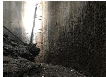
were run from a generator located on the ground. As operatives broke out each section of concrete wall, the sections were lifted out and deposited down a rubble chute positioned on the scaffold - this allowed the material to be removed from site efficiently.
