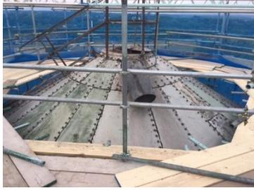
Once the scaffolding had been erected, one of Lawson Group's highly trained demolition supervisors assessed the scaffolding up to the top of the silo. Once confident that the scaffolding met Lawson Group's high standards, cutting of the metal roof could begin. Using a disc cutter, sections were cut out and allowed to fall, in a controlled manner, into the pre-determined drop zone within the silo.
