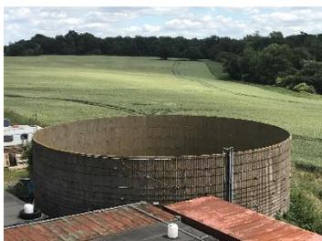
Both silos were constructed of the same material - pre-cast panels with post tensioned hoop bars fixed externally.
