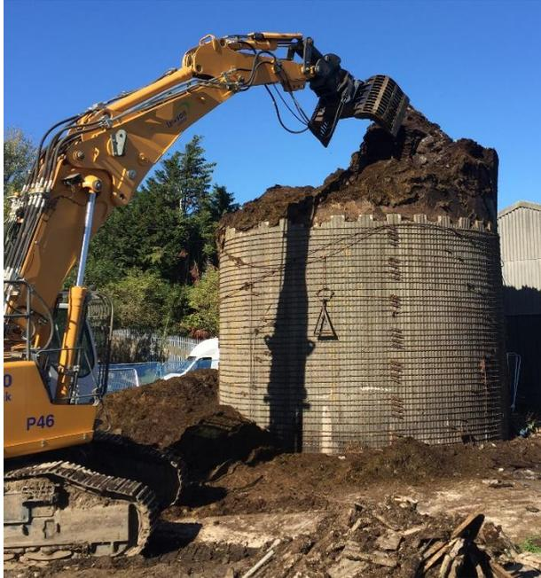
Due to the rotted and wet straw located inside the silo, the hand demolition process could only proceed down to approximately eight and a half metres from the ground floor. At this point the scaffold tower was carefully removed.
