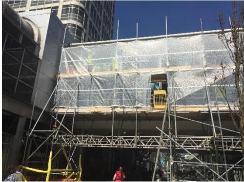
A tower scaffold was used to access the underside of the ceiling. The plaster board was lightly wetted to minimise any dust generated, the ceiling was then removed and lowered to ground level. All M&E was cut out and removed, as each area of work was completed it was inspected by the site supervisor to ensure all loose material had been removed.
