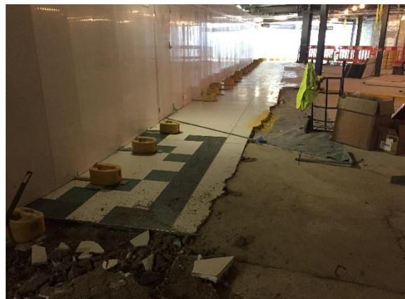
across. Using floor scrapers, the floor tiles were quietly lifted. As each section was removed, they were loaded into a wheelbarrow and removed via the goods lift.
