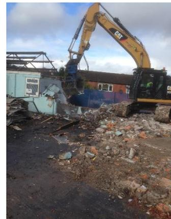
Once the roof had been safely removed the deconstruction and crushing of the building could begin. This was carried out using a similar method to that described above for Broomhill House.
