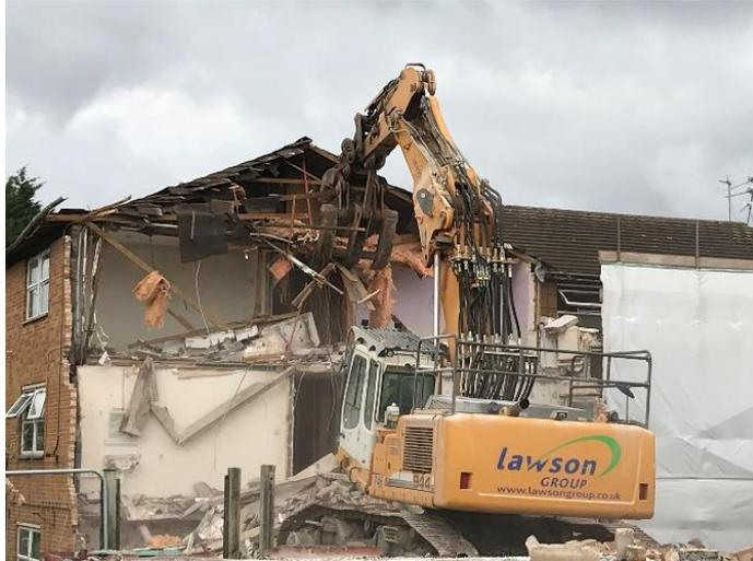
Using a hydraulic grab attachment, the roof was removed back to the first supporting column allowing one bay of the roof to be lowered carefully to the ground floor slab. The wood and timber sections were then removed and lowered to ground level, away from the building and were later processed and loaded into the designated forty-yard waste bins. Once the roof had been removed, the internal walls and floors were removed and lowered to ground level.
