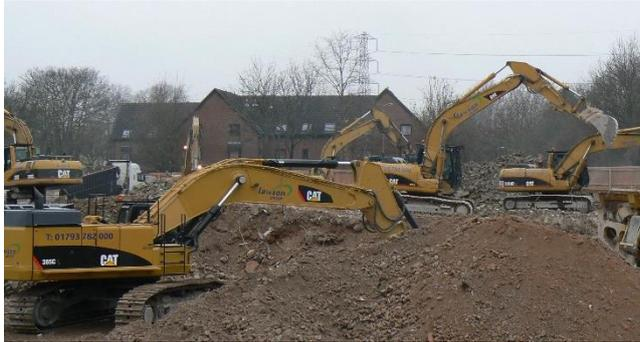
The remainder of ground floor slab was broken onto the basement slab. Walls and columns in the basement were then reduced to 150mm above the existing adjacent ground bearing slabs. Plant working in the basements were provided with a minimum 600mm mat of demolition debris or crushed concrete laid over the slab as protection.
