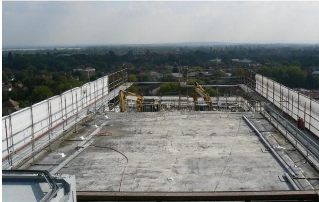
Only with the above activities completed or in place could demolition work commence of the existing structure. To facilitate demolition of the structure, up to 13T 360° excavators and 3 tonne bobcats were lifted to roof level and onto the 9th floor slab using a mobile crane.
