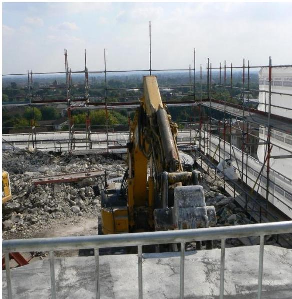
This progressive small machine demolition involved the use of up to 13-tonne excavators, equipped with either pneumatic pulverisers or breakers which undertook progressive small machine demolition. Due to weight restrictions, only one machine could be used in any one bay, at any given time (a bay being a floor area usually between four existing columns).
