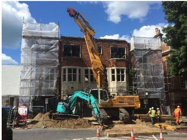
Due to the close proximity of neighbouring properties the gable end was removed by hand. Access scaffolding was erected to the side and fitted with handrails and Monoflex. Drop zones were created inside the building to prevent debris spreading.
