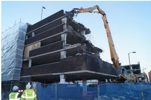
had been reduced. The arisings generated from the demolition were utilised to form a ramp for the high reach excavator to use as a platform to work on in order to reach the remaining high-level lift motor rooms and stairwells. Steel elements of the building were mechanically cut with a hydraulic shear attachment and were lowered to ground level.
