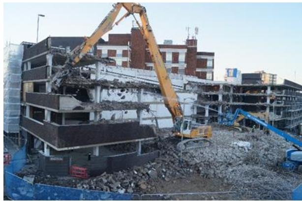
Throughout this process the demolition excavator operator ensured that the structural support elements remained in situ until all other structures that took such supports, like the shear walls,
