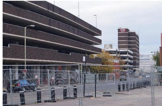
**SOLUTION:** An initial soft strip was required as part of the preparation of the multi-storey car park, however this was minimal due to the nature of an open plan multi-storey car park which consisted mainly of open floor space. The main areas which required a more thorough soft strip were the stairwells and shop mobility areas.
