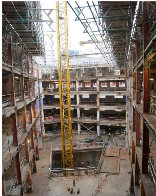
**RESULT:** 95% of the materials from the soft strip and structural demolition were recycled as most of the debris consisted of steel and concrete. The 1930's art deco building had been given a new lease of life as it was to be transformed into luxury apartments and penthouses.
