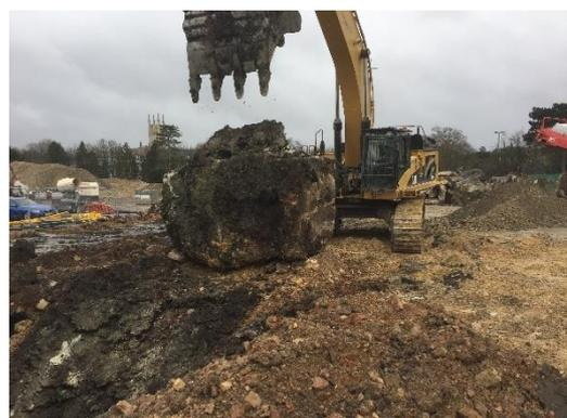
excavator returned to the edge of the slab and dug around the first foundation.
