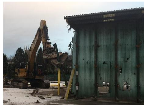
Using the hydraulic sheer attachment, the roof purling's were cut back to the next supporting roof beam allowing.
