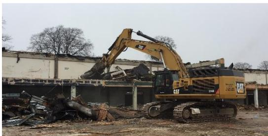
The demolition excavator then removed the concrete frame, generated from the above process, and stockpiled away from the working area. Each piece of steel and concrete was thoroughly inspected for any remaining asbestos cement.
