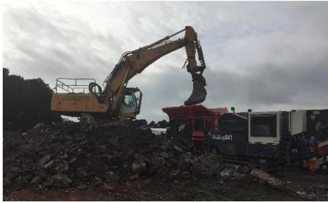
The foundation was lifted out and stockpiled ready for breaking. The area of ground from where the foundation had been removed was then back filled and tracked in. This process was repeated until all foundations had been removed. Once a stockpile of concrete had been generated, a second excavator with breaker attachment then proceeded to break the concrete into pieces no bigger than 500cm<sup>2</sup>. The Mobile Crusher was operated in accordance with the Safe
