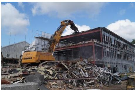
Lawson Group's own Liebherr 954 was used with a multiprocessor shear attachment to demolish the remaining structure. Works then commenced at the Eastern elevation.
