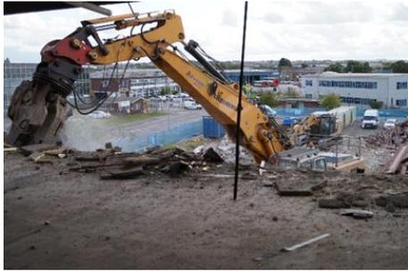
throughout the remaining structure. Dust suppression was maintained throughout the works by means of a Dustboss.
