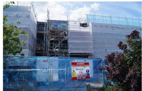
First and second floor areas were serviced and accessed via a HAKI staircase with bag and airlocks positioned on the scaffold platforms. Waste and transit routes from upper floors were also via a HAKI staircase. This transit route was an exclusion zone and access was prohibited for any other site operations. An enclosure was formed to remove the AIB boxing to service ducts, cladding to steel beams and columns, fire breaks and panels above and below windows.
