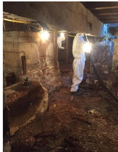
**SOLUTION:** All the loose AIB debris and AIB panels were carefully removed and bagged immediately. When the AIB was too big to bag, it was double wrapped in 1,000-gauge polythene, red bags and marked accordingly.
