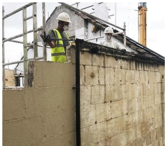
The tower scaffold was relocated to the ground floor, the first-floor floorboards and timbers were then cut out using reciprocating saws and removed from the building. Much of the work on the ground floor continued in a similar vein to that previously above.
