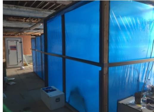
Prior to dismantling the enclosure, an independent analyst carried out a four-stage clearance. After the analyst had passed the visual and air tests, operatives then proceeded to take down the enclosure and bag the 1,000-gauge polythene as waste. This was double-bagged and carefully disposed of as asbestos waste.
