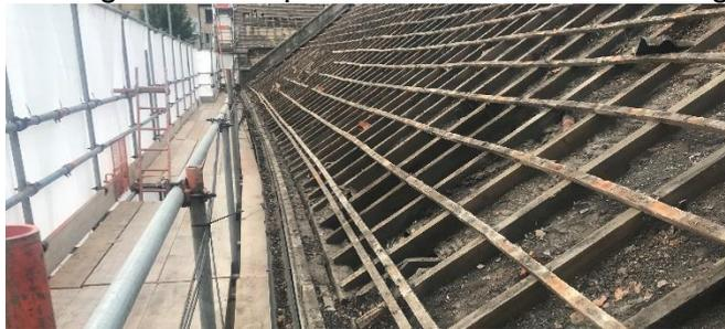
plywood sheets were laid on the timber floor for protection. Using a tower scaffold for access to the building, the operatives started removing the roof tiles and timbers. The tiles were passed to operatives on the first floor and were stacked on the scaffold ready for removal. Care was taken not to overload the scaffolding. Once the roof tiles had
