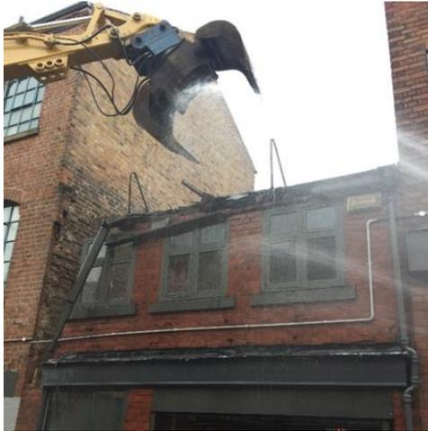
All services were terminated and disconnected before demolition works commenced. Before any mechanical demolition works could take place, buildings were soft stripped of all loose fixtures and fittings. Scaffolding was erected and hand separation was completed. A dust boss was used to suppress dust, providing a blanket screen of water over a demolition zone to protect the surrounding environment.
