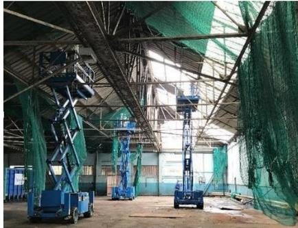
(MEWPs) to remove the sheets. Three MEWPs were in operation with a pair of operatives assigned to each one, all operatives were IPAF and CAT B trained. MEWPs were logistically positioned for the safe removal of CBA sheets. All sheets were first dampened using a suppressant mix, the bolts were cut and sheets lowered one by one. They were then removed using a skid steer and placed in a stacked pile into an enclosed 40-yard skip. During the CBA
