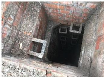
Included in the scope of works was the requirement to remove all footings, slab and hard standings. Due to the previous use of the site, several manholes were located within the site boundary - this was a challenging element of the project.
