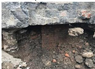
surrounding the manhole were removed, the access was raised and encroached above ground level. Lawson Group were required to reduce the height whilst protecting the Wessex Water's assets below ground. Confined space trained operatives installed a scaffold crash deck to prevent any falling debris. The surrounding piles
