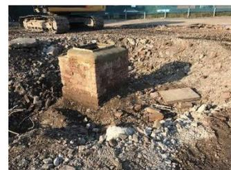
Additional requirements within the scope included the instruction to locate and remove all obstructions up to 3m deep, this included the removal of 1no Interceptor tanks and 2no storage tanks. Lawson Group were required to plot on drawings where remaining piles footings were left that exceeded a depth of 3 metres.
