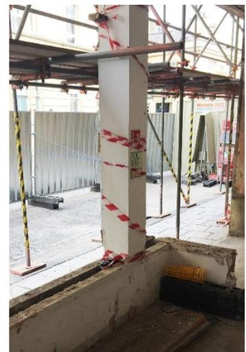
wrapped at this stage. Operatives accessed the high level AIB by using a small podium and used the same process as per the lower level methodology.
