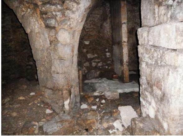
The basement also needed to be removed in this part of the building. This was hand dug and using a conveyor belt, spoil was moved up to the ground floor where it was transported to a 20-yard skip via small power dumpers.
