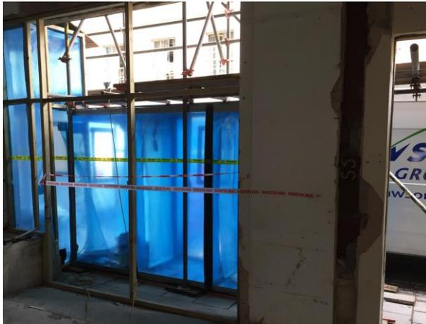
As panels were removed, the voids were inspected for any apertures to adjoining areas and were sealed as necessary. All visible dust and/or debris/cobwebs etc. within brickwork cavity and the enclosure were wiped clean or vacuumed using a Class H vacuum cleaner. Standard operating procedures were followed for decontamination, waste removal and four stage air clearance.
