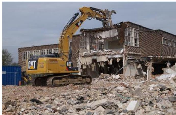
**RESULT:** All slab, foundations and underground obstructions were removed, all concrete and hard-core were processed on site producing 6f2 crushed stone material suitable for recycling within the future residential development. The project was completed to programme and to the client's specifications and successfully handed over.
