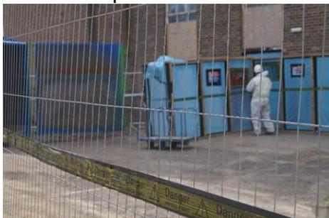
Lawson Environmental's qualified operatives undertook the enabling works to erect negative pressure enclosures. These were smoke tested to ensure bag,
