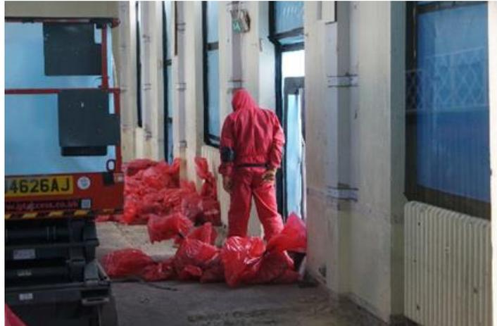
Full floor to ceiling enclosures were erected, a MEWP was lined with polythene and used for access to reach the AIB panels. These were dampened using a low-pressure sprayer from the underside. Once wet, the nails were removed ensuring the panel remained whole whilst being lowered to the ground. The panels were then double wrapped and bagged in waste bags marked as hazardous.
