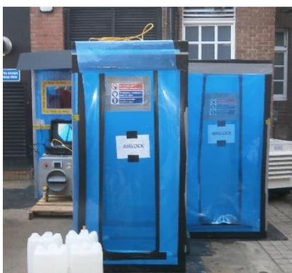
The Kitchener Hall Boiler Room (Licensed work) required the setup of airlocks, constructed out of 1,000-gauge polythene on a metal tube frame standing 2m high.
