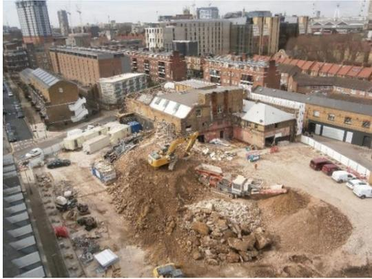
The works commenced with licensed asbestos removal undertaken by Lawson Environmental (part of Lawson Group). The licensed asbestos was detected in a Refurbishment and Demolition Survey which found asbestos in multiple areas of the site. Approved plans of work were implemented detailing confined space works for asbestos removal within basements and ducting voids.
