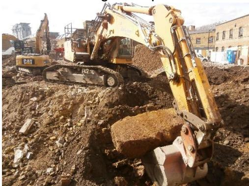
Lawson Group offers most clients as they are licensed to crush demolition arisings to a 6F2 specification which allows the clients to use the crushed material as a sub base for roads.
