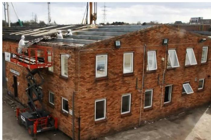
Once the soft strip and asbestos removal had been completed to the satisfaction of the site supervisor then the mechanical demolition of the structures could begin.
