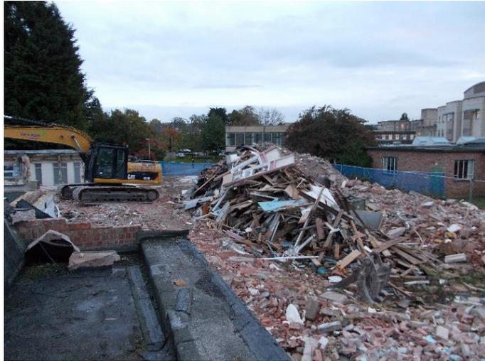
Hand separation was utilised on the retained corridor of the site and the tower next to it.
