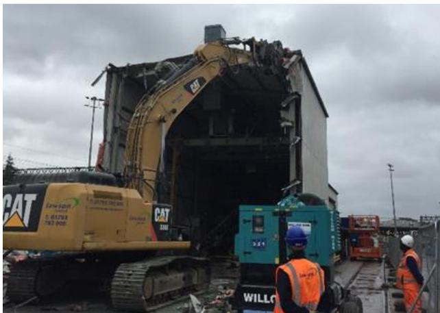
The environment was protected by utilising a Dust boss that produces a fine mist suppressing the release of any dust. Noise monitoring was carried out during works to ensure exposure levels were not exceeded.
