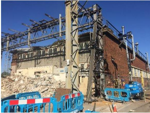
was loaded and carted away utilising the onsite rail infrastructure. Height restriction barriers were placed at all site entry points and each demolition zone was detained within solid timber hoarding.
