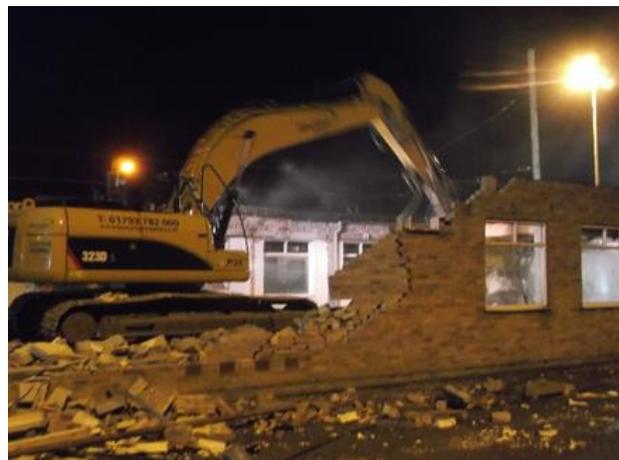
Due to the live operation of the rail depot shift patterns, night works were required. Temporary lighting was installed and demolition works continued throughout night time shifts. All deliveries and traffic movements were
