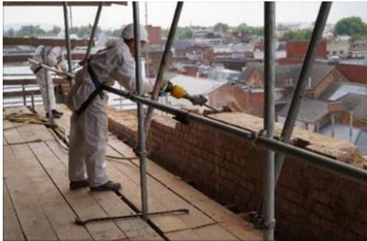
Lawson Environmental (part of Lawson Group) were used to remove the asbestos from the premises in order to allow for a safe demolition to start. Demolition began with the old main dealer garage and the surrounding forecourt. The methodology was simple and tailored to suit the showroom building, the forecourt area and the collection car park.
