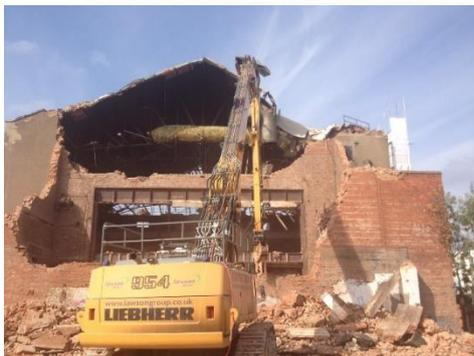
A Liebherr high reach excavator was used with a four-tonne scissor attachment to demolish the skeleton of the building. Work commenced at the back and worked forwards towards the front hand-demolished wall. Using this machine allowed for the demolition of the framework to be controlled, firstly breaking through the brick work to reveal the architecture of the large theatre.
