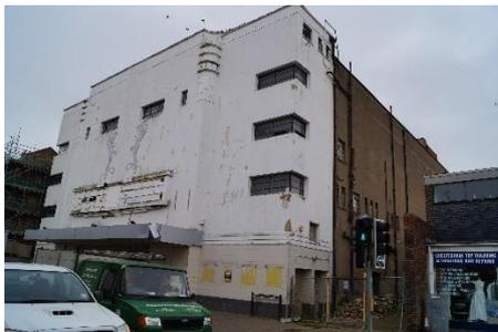
As a result of an asbestos survey, licenced asbestos was found in the cinema and non-licenced asbestos was found in both the cinema and the garage. Images of two ladies, entwined in celluloid on the front of the cinema, had to be removed in such away so that they could be salvaged and placed on display at another site.
