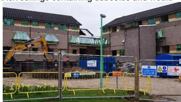
**SOLUTION:** Before any work could commence, bat boxes had to be erected in close proximity to the site in accordance with the site's ecology report. As per the agreed plan, each of the two blocks underwent soft stripping to remove all non-fixed and loose waste. Secure drop zones were created in order to ensure the safety of the operatives and separation of the waste products.
