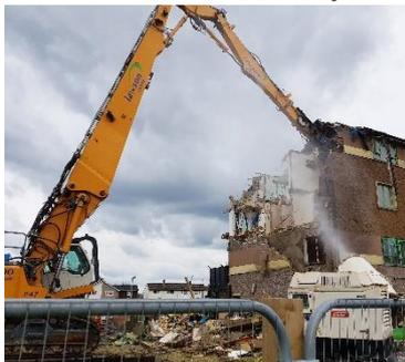
Block A was stripped first so non-licensed asbestos, including that found in the Artex, could be removed whilst soft stripping was taking place in Block B. Artex ceilings were carefully
