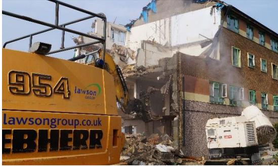
removed, the waste was double-bagged and sealed ready for safe disposal. Only when all the loose waste and asbestos had been removed could mechanical demolition start on the two main residential blocks.
