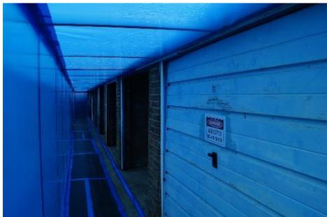
As one of the two separate garage blocks was found to contain licensed asbestos, the works were notified to the HSE with an ASB5. The garages were sealed and completed under controlled conditions by Lawson Environmental (part of Lawson Group) whom are licensed by the HSE to work with asbestos. Only when the asbestos had been removed, by Lawson Environmental's highly trained operatives, could the mechanical demolition on the garage blocks begin.
