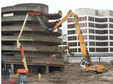
**RESULT:** At the end of each of the phases, the demolition arisings were crushed on site to a 6F2 specification so that they could be reused on site for the redevelopment. Lawson Group anticipated recycling 100% of the waste generated at Carlton Street multi-storey car park. This target was reached as the materials within the build consisted of concrete and steel.
