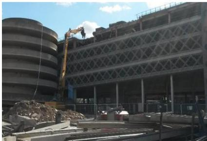
The second phase of works were between grid lines 1-2 M-F, again commencing on the fifth floor and working progressively
