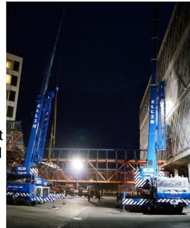
**SOLUTION:** The bridge was removed under a contracted lift which required two cranes to lift and lower the 36-tonne bridge to ground level. After the successful removal of the footbridge,
