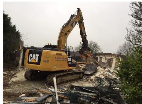
Once the roof had been removed on each building, the grab was positioned over the top of the wall, each grab was lowered to ground level. A handheld killer sprayer was used to wet the brick and any asbestos cement products that were present. A fully trained operative carefully moved each brick and picked out pieces of asbestos and placed them in asbestos bags.
