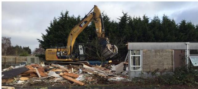
Loose contents from within the structures, including furniture, appliances and general waste were removed by hand in a controlled manner and arisings managed in accordance with the Site Waste Management Plan. Door frames and skirting boards were removed by using bar and sledge hammers. Only operatives
