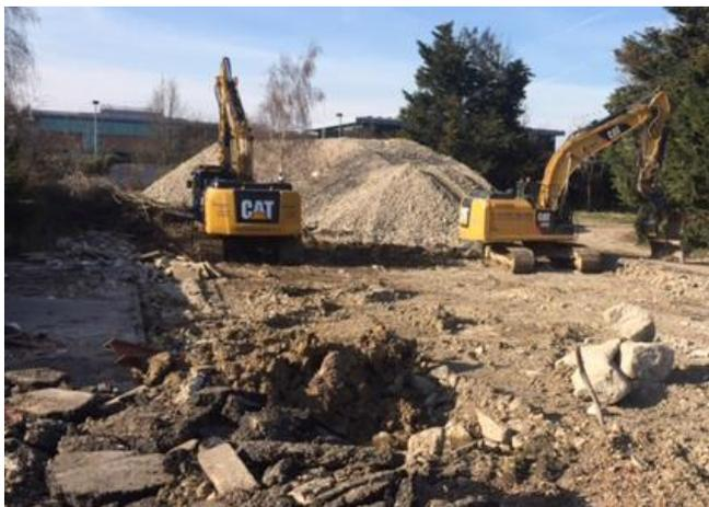
Throughout the demolition process, Dust bosses were used for dust suppression to ensure environmental expectations were met. A crusher was used to process the arisings to a specification as agreed with the client.
