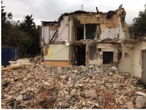
frames, skirting, suspended ceilings, floor coverings and plasterboard timber partitions. All materials were removed in a controlled manner and segregated.
