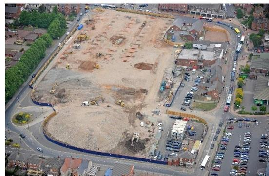
**RESULT:** All loose fixtures and fittings were removed and segregated for recycling or disposal. The foundations and ground floor slab were excavated to 1.5m to leave site clear. The works were completed on time and within budget. The site was handed back to the client ready for the next stage of the new store development.
