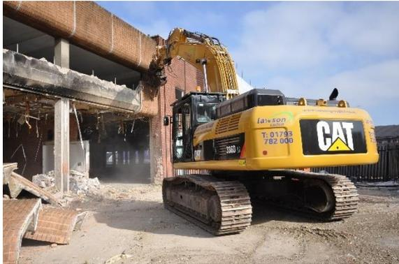
demolition then commenced, starting with the former car repair garage and the residential properties located on the perimeter of the site. The Swan pub was then demolished in a similar manner, with extra care being taken in the demolition due to the close proximity of the structure to the main road and pedestrian walkway.
